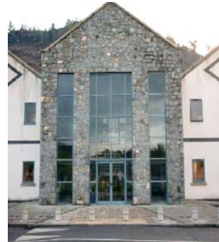
Branas Isaf Offices – Corwen, north Wales
